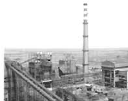
Captive Power Plant
