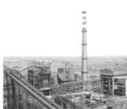
Captive Power Plant
